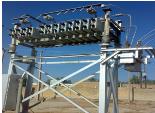
Figure 3 Capacitor bank of a power station of the regional power dispatching company of Khuzestan (South-West Iran).
