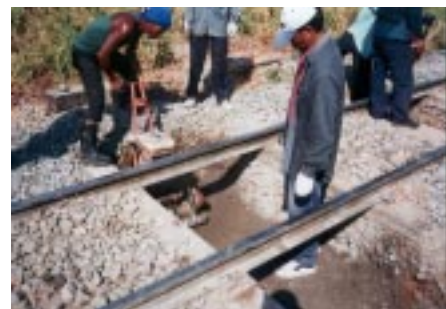
Figure 16 Compaction of test embankment
