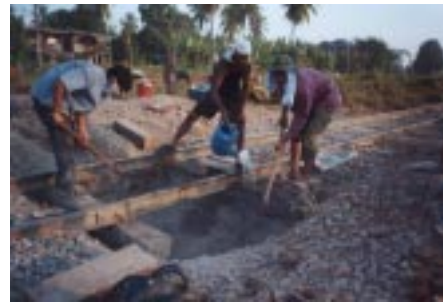
Figure 15 Mixing and Placing tested embankment
