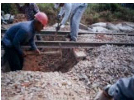
Figure 12 Removing of existing embankment
