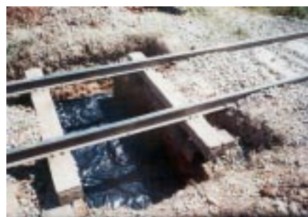
Figure 14 Placing of Plastic sheet to prevent moisture from original ground
