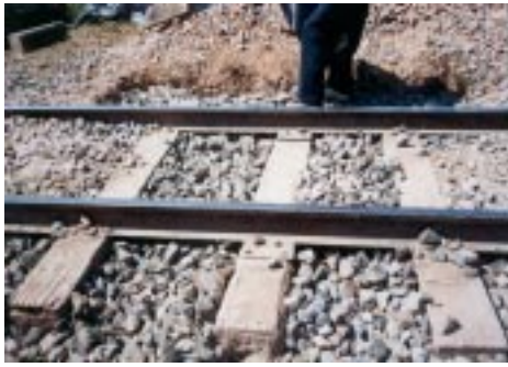
Figure 17 Completed test embankment
