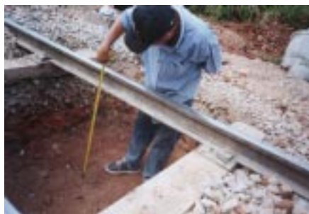
Figure 13 Depth checking before embankment Construction
