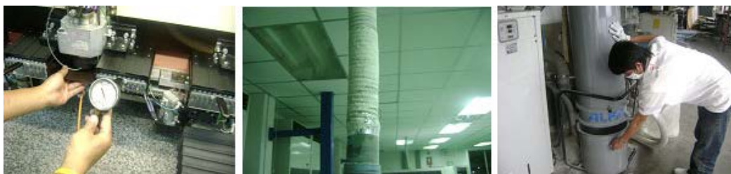
Figure 4 Vacuum test, vacuum tube and dust bag inspection
