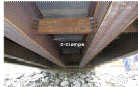
Figure 12. Deck-Stringer Connections with Z-Clamps
