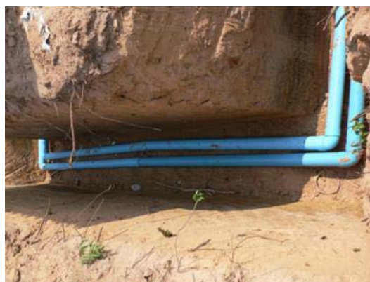
Figure 4. Installation of earth-to-air heat exchanger
