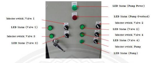
Figure 4 Control panel of the control box
