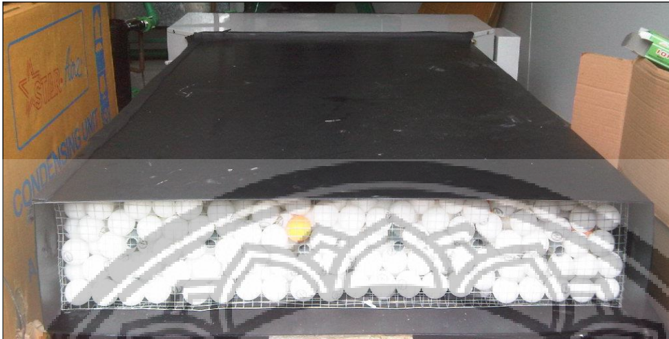
Figure 4 Installing the PCM bed in the return duct.
