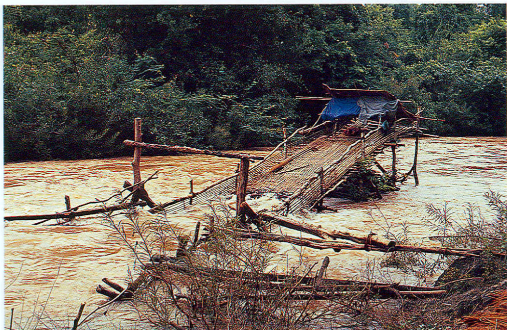
Figure 11. It takes about a month to build a single li trap out of wood, bamboo, rattan, vines and sometimes nails in the Khone Falls area.
