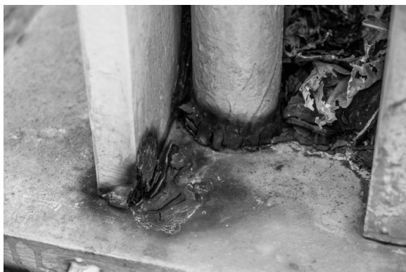
Fig. 4 Corrosion at weld of the column in power plant
