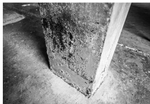
Fig. 2 Corrosion on the steel column in power plant
