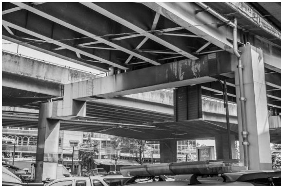
Fig. 5 Steel expressway with deteriorated coating
