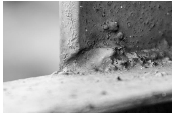
Fig. 6 Undercut at the weld on steel billboard
