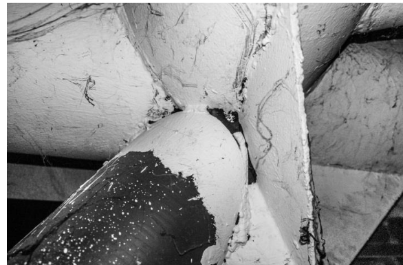
Fig. 9 Discontinuity of weld on steel pipe roof structure
