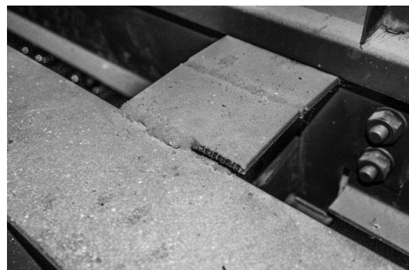
Fig. 10 Missing weld on steel beam girder
