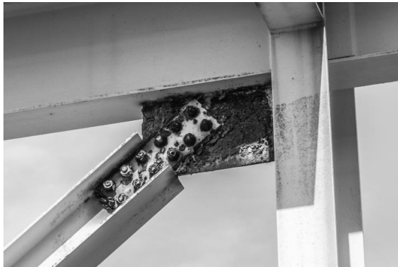
Fig. 3 Corrosion at steel bolt and plate in power plant
