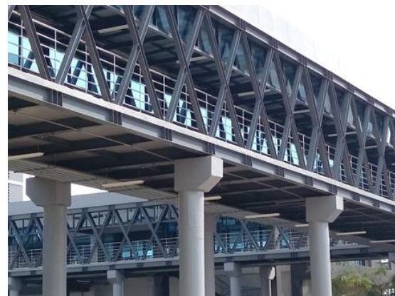
Figure 1 A pedestrian bridge supported on RC corbels at Khon Kaen University
