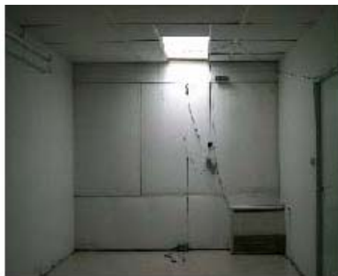
Fig. 6 Picture of interior space of the experimental room at 9.00am on 7 July 2004
